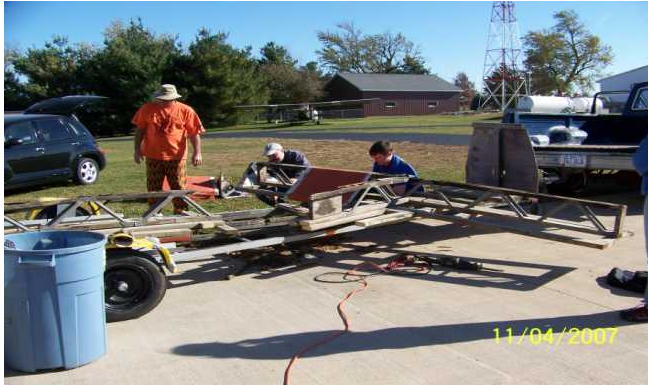
Volunteers 'deconstruct' the old wind tee.
