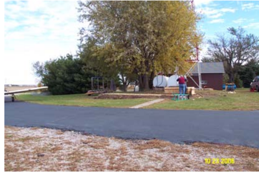
Rod Thompson and Bill Crippen build the forms.
